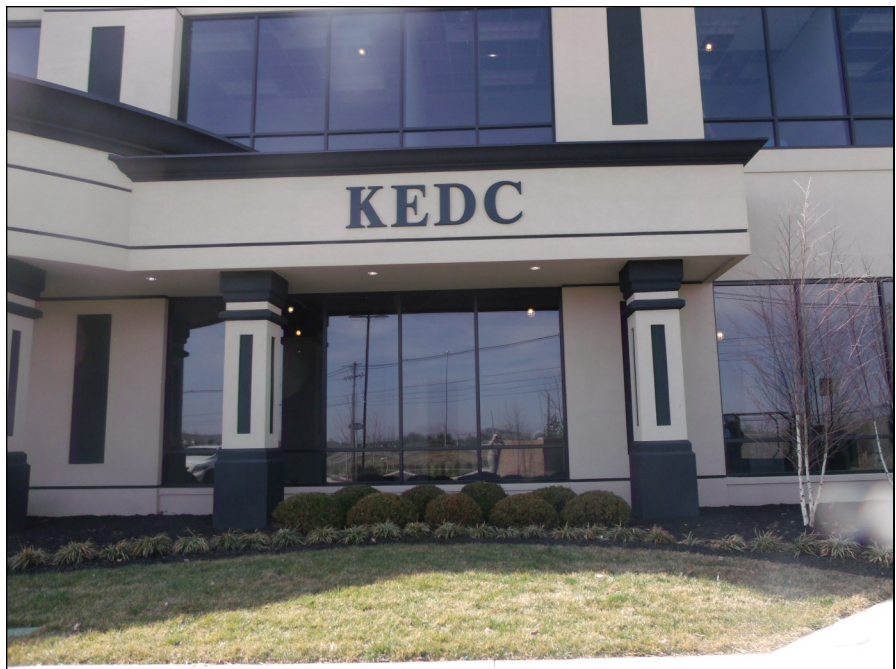
KEDC Lexington Office and Conference Center
