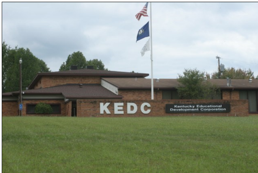
KEDC Ashland Office and Conference Center
